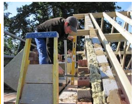
(Aaron Laying a brick)
